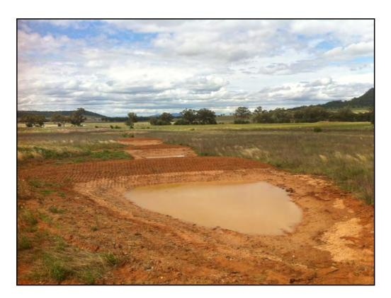
Plate 1 – Newly constructed sediment traps 30/11/2011
